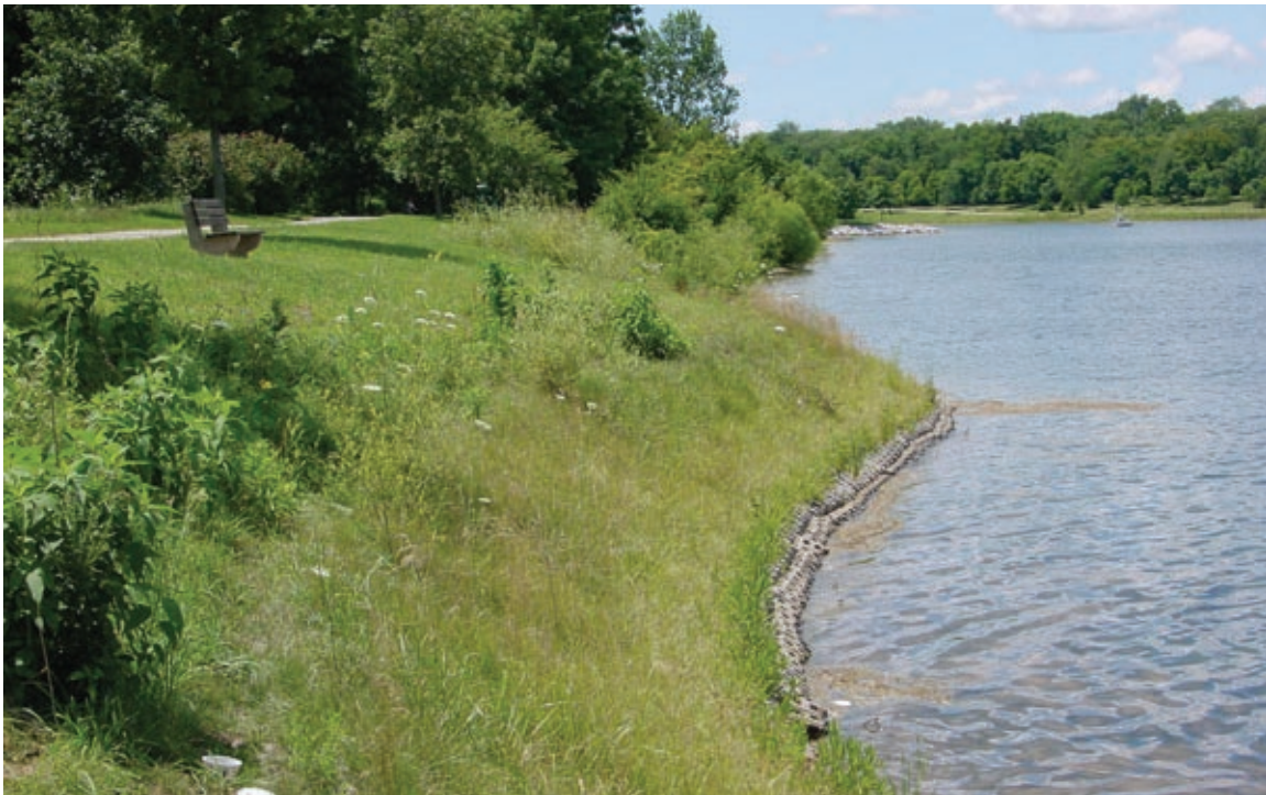
Example photo of a fully vegetated articulated concrete block/geotextile installation
