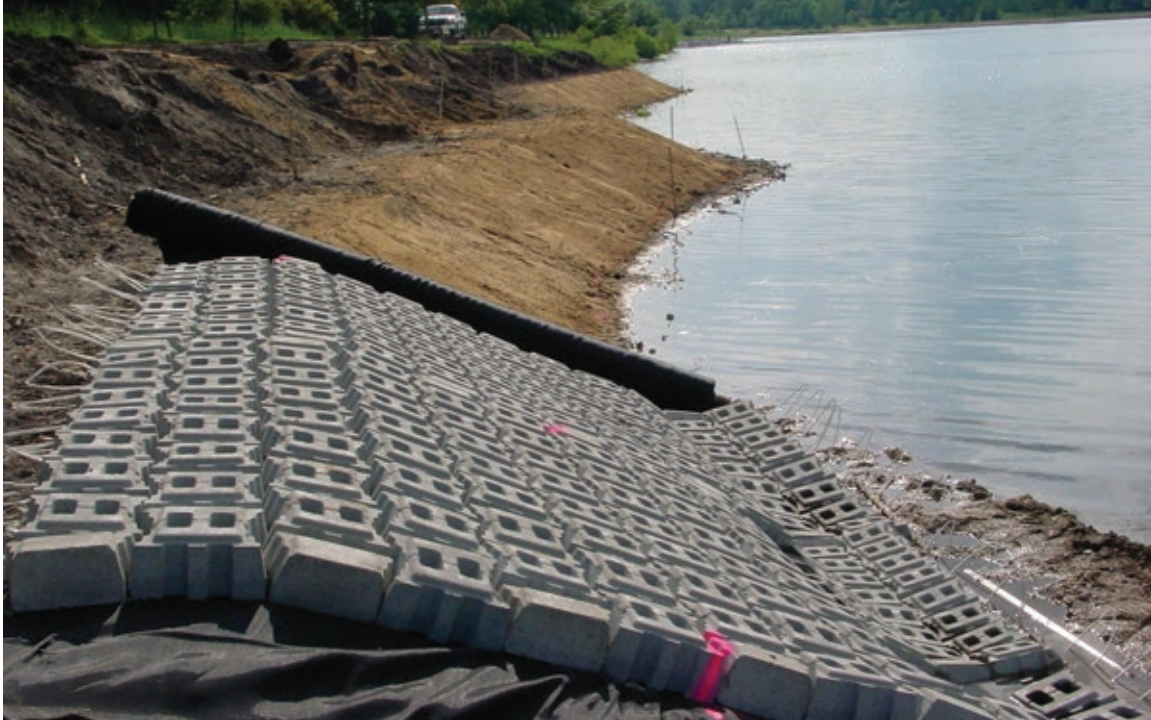
Example photo of articulated concrete block installation with geotextile/filter fabric
