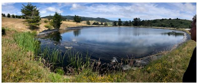
This picture shows the 10 AF pond to be lined with a poly-liner. The black material on the edges of the pond currently is being used for vegetation management and is not lining used for waterproofing the pond berms.
