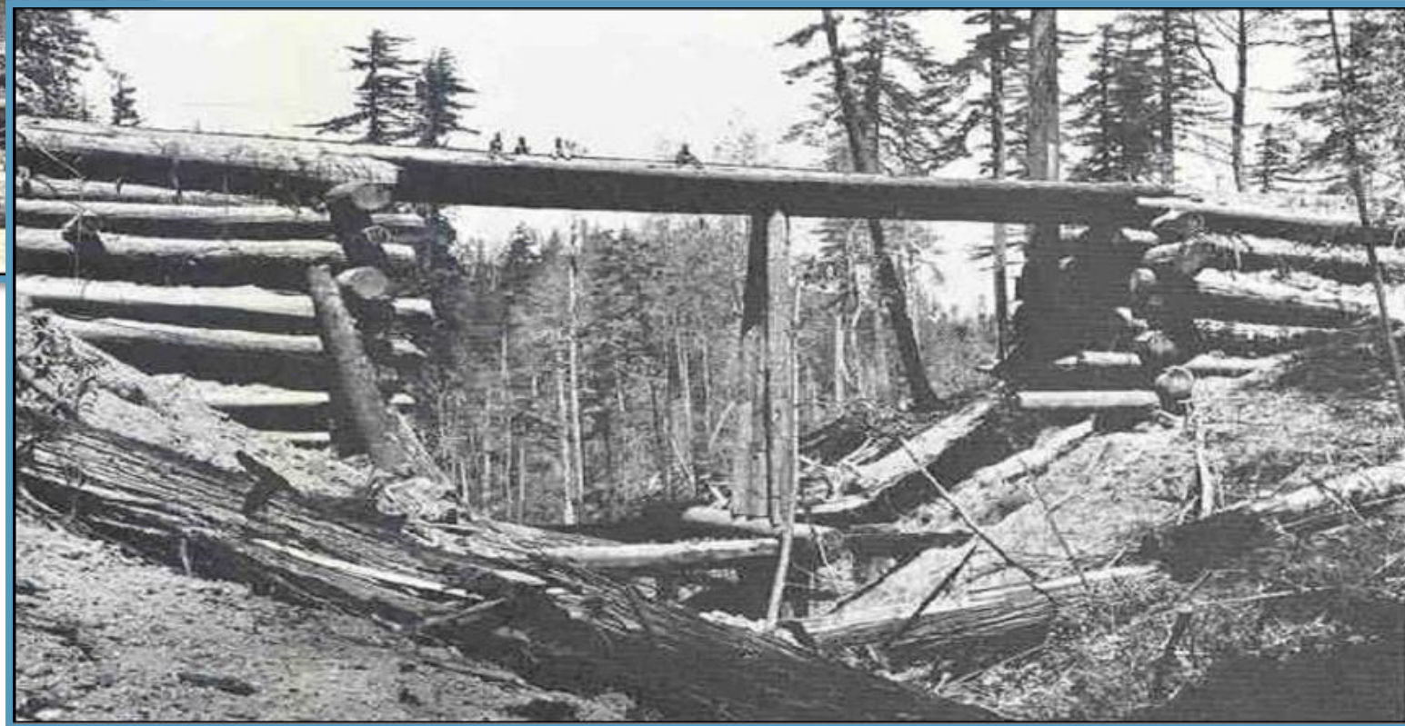
Crib log, or “Humbolt,” creek crossing on Old Haul Road. Note the men sitting on top of the crossing. Photo: Santa Cruz Lumber Company (1943)
