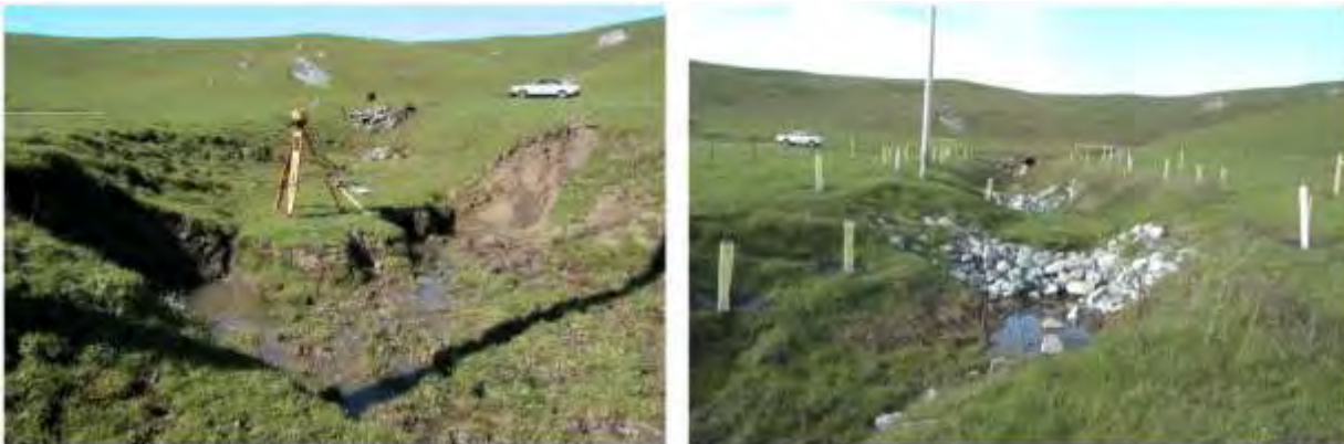
Rock chutes. Treatment of gully with rock chutes. During installation (left) and after (right) (from Marin RCD). In this treatment only the steep scarps of the gully were treated. In some areas the entire gully may need to be armored, requiring substantial quantities of rock
