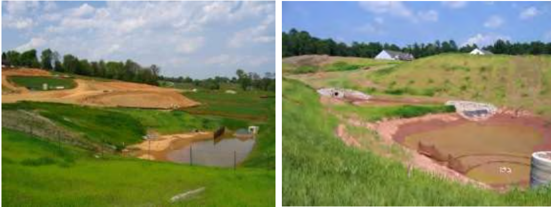
Sediment catch basin. Examples of sediment catch basins. The site drains to pond so that sediment can settle before water is allowed to discharge into nearby creeks.
