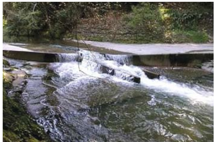
Above: The completed vehicle ford with pre-cast arched culverts to allow freer passage for fish. Right: The vehicle ford before being torn down and replaced. Photo credit: San Mateo RCD
