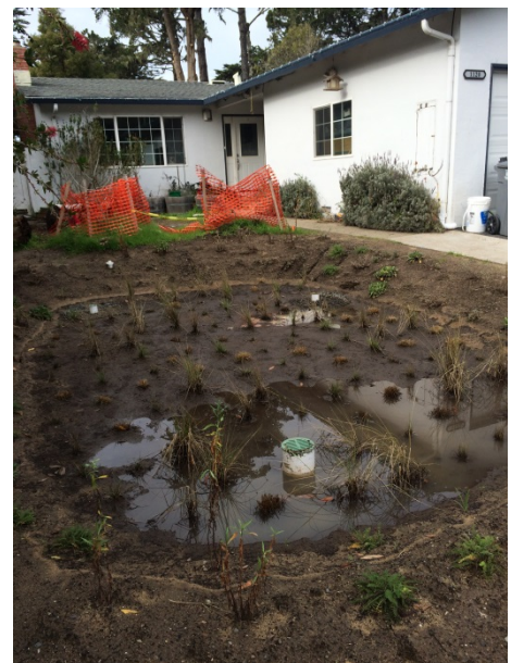
Rain garden during construction, Montara
