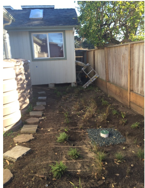
Completed rainwater harvesting and rain garden system, Moss Beach
