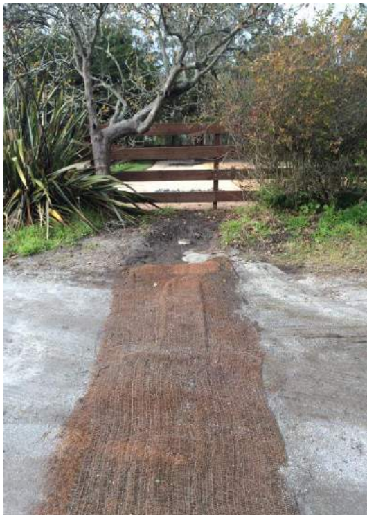
Installing drainage road inlet with temporary erosion control mats leading to the bioswale
