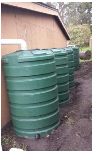
Rain barrels with first flush system
