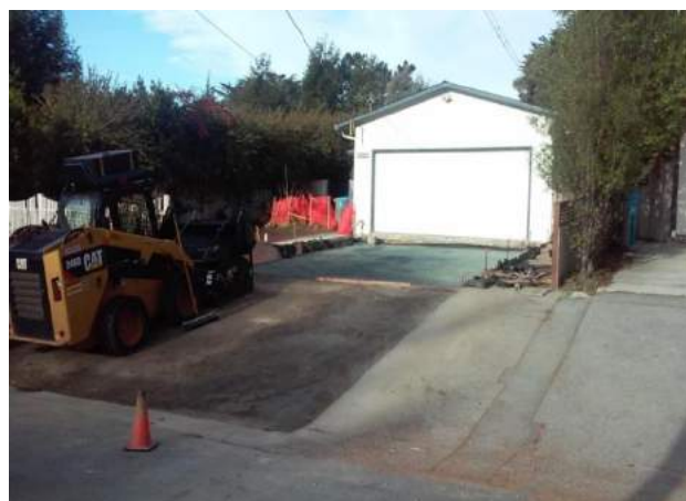
Installation of asphalt driveway with permeable section on top and regular asphalt on bottom
