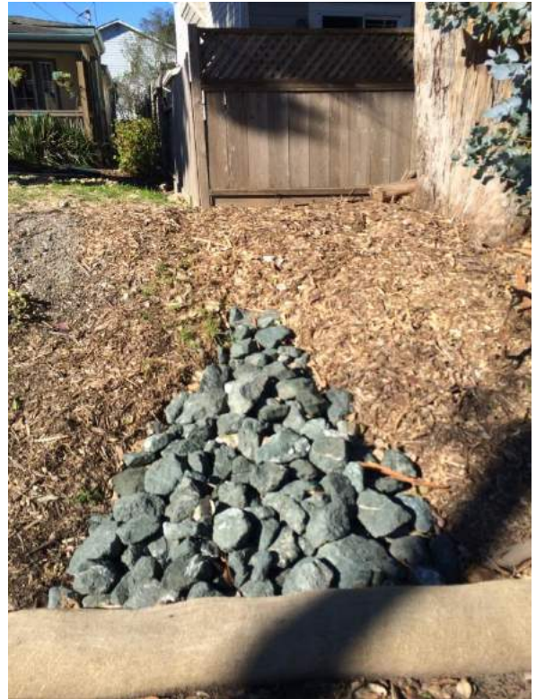
South side of property with drain line under rock (left) leading to gravel drainage outlet with riprap (right)
