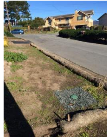
Permeable asphalt driveway (left) and underdrain and outlet for driveway (right)
