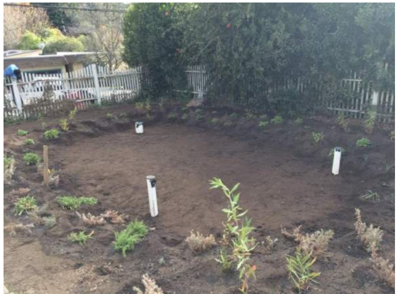
Installation of rain garden
