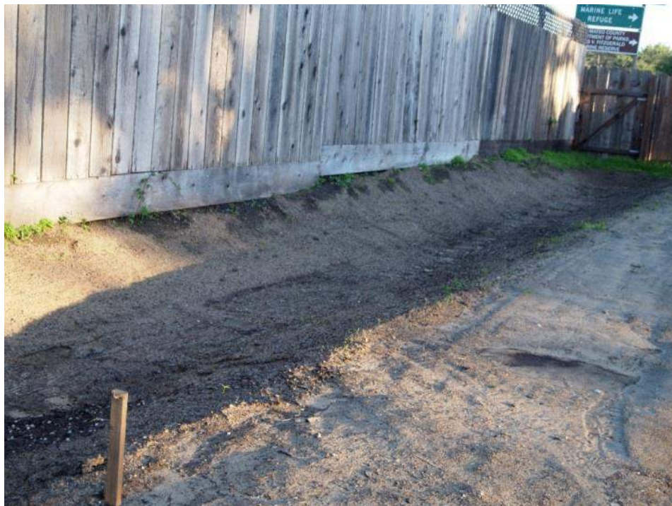
Filling in trench with biosoil mix
