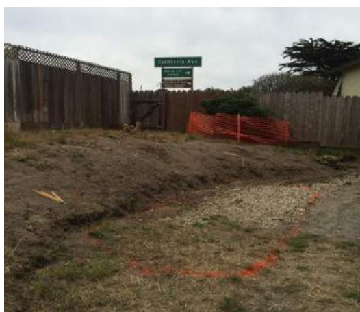
Marking site of eastern rain garden
