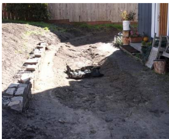
Digging eastern rain garden
