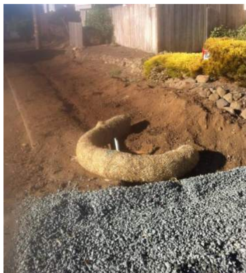
South side of property showing driveway underdrain and outlet area
