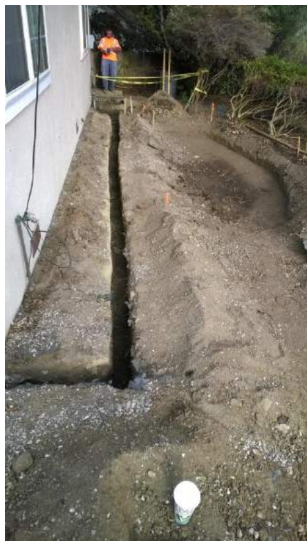
Piping from downspouts to rain garden
