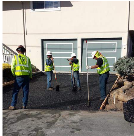
South side of property showing permeable asphalt work on driveway
