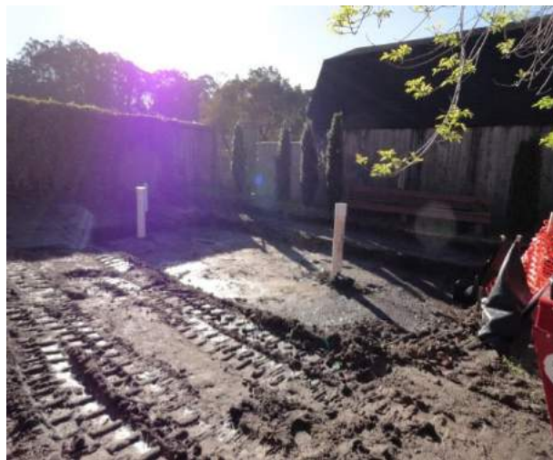
Grading of rain garden and piping installation
