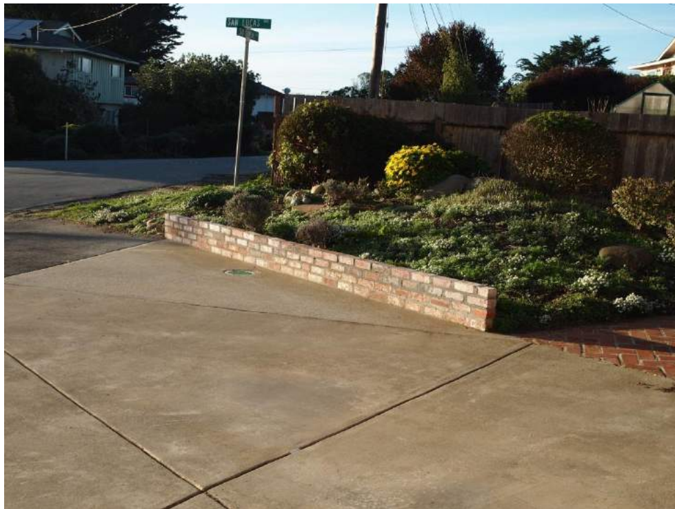
West side of property showing new brick wall/erosion control structure
