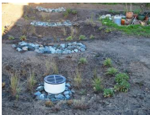
Native plants including grasses, sedges and natives within the three-pooled rain garden system
