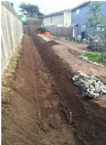
Marking and digging trench for bioswale
