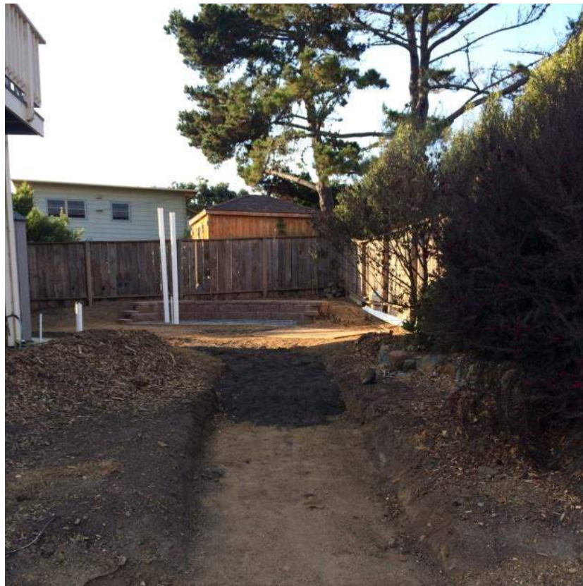
Upstream section of the bioswale/rain garden system
