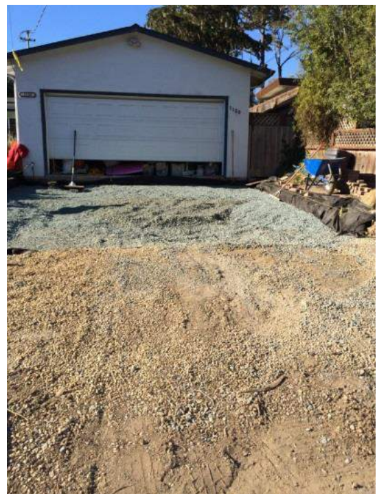
Removal of concrete driveway and installation of base layers
