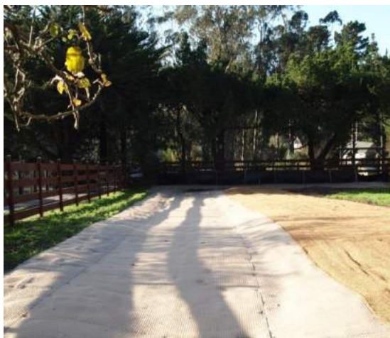
Turf reinforcement mat placed in graded swale area and temporary erosion control mats
