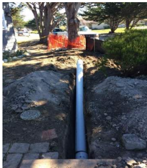
Laying pipe alongside house from three-tiered rain garden towards west rain garden
