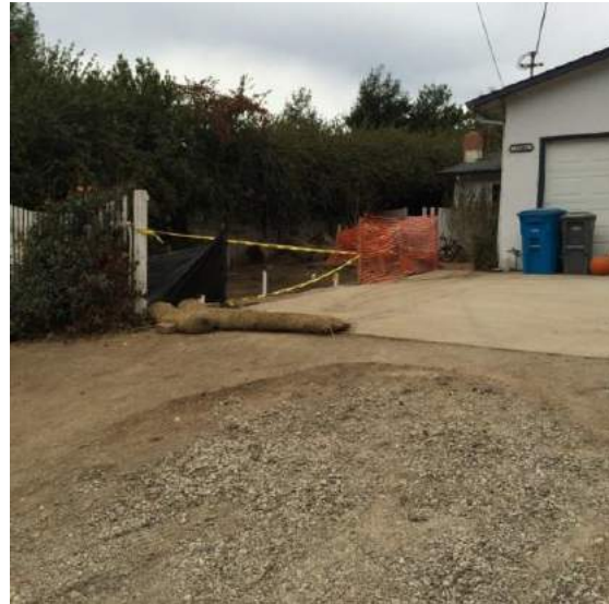
Stump removal from driveway
