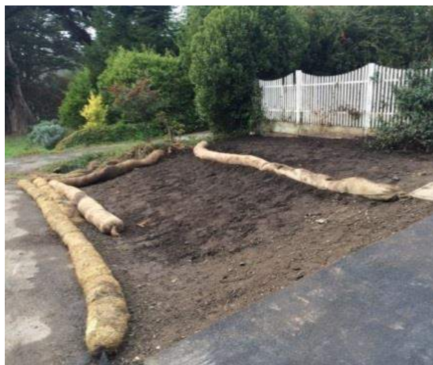
Side driveway area with asphalt removed and erosion control mats installed for vegetation
