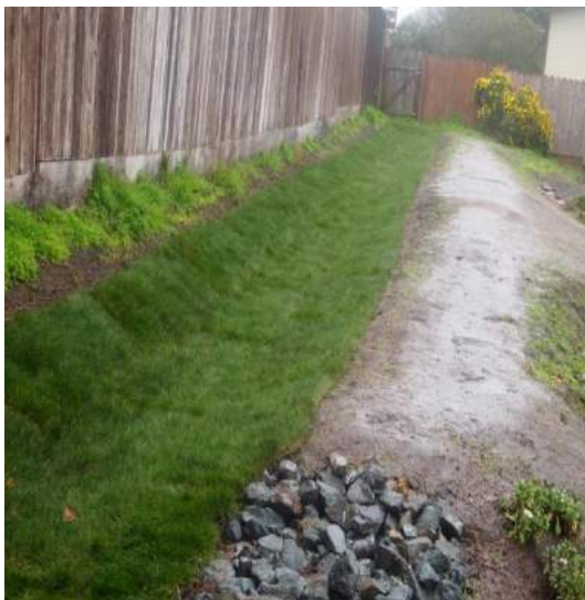
Bioswale of native no-mow grass to collect runoff from the adjacent public highway
