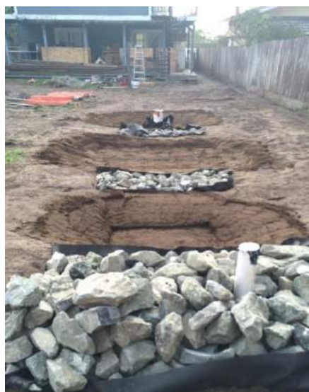
Shaping the three basins of the three-tiered rain garden showing outlet riser and rock weirs
