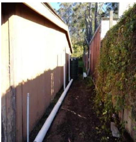
Installations of rain barrels with overflow drain line leading to rain garden
