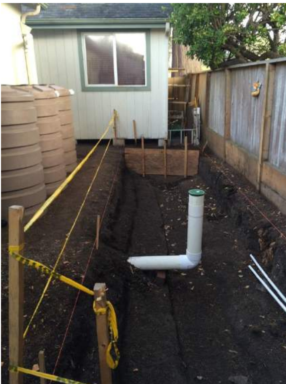
Installation of rain water tanks and rain garden on south side of house
