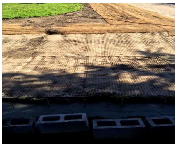
Installation of overflow weirs
