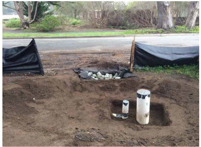
Piping for roof runoff and leading to western rain garden
