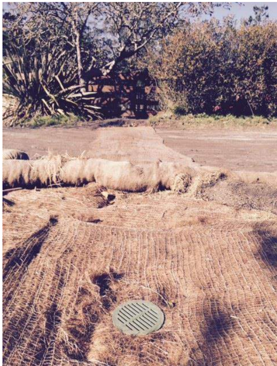
Installing drainage road inlet with temporary erosion control mats leading to the bioswale
