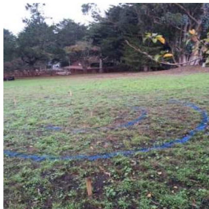
Marking of bioswale
