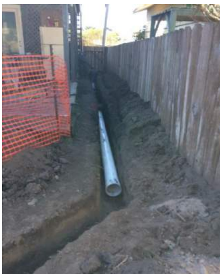
Laying pipe alongside house from three-tiered rain garden towards west rain garden
