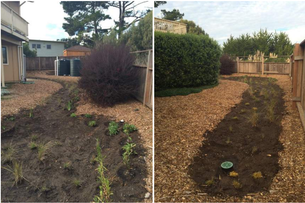
Bioswale/rain garden system
