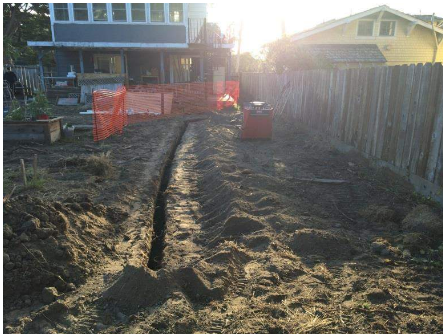
Trenching for pipes beneath the three-tiered rain garden
