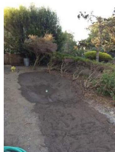
Rain garden area where tree was removed (left), bioswale leading to the rain garden (middle), and bioswale to rain garden connection
