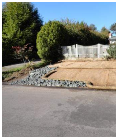
Side driveway area with asphalt removed and erosion control mats installed for vegetation
