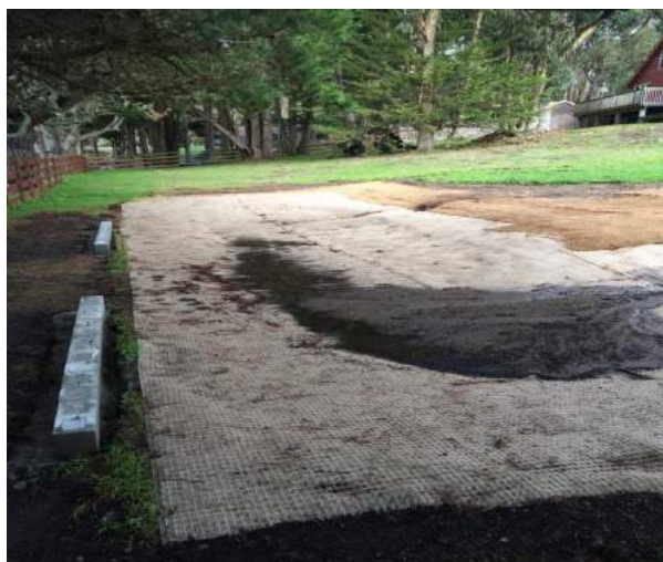
Overflow weirs located at the bottom of the bioswale
