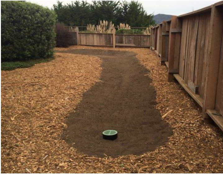
Downstream section of bioswale/rain garden system
