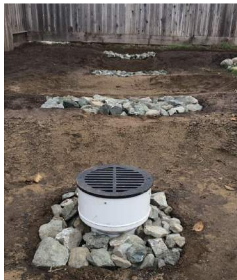
Shaping the three basins of the three-tiered rain garden showing outlet riser and rock weirs
