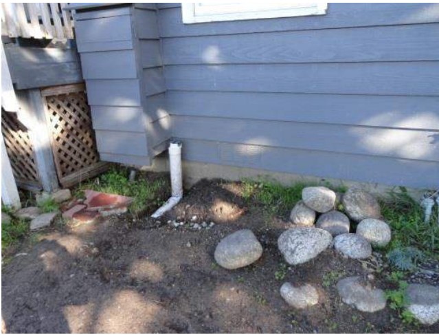
Piping for roof runoff and leading to western rain garden
