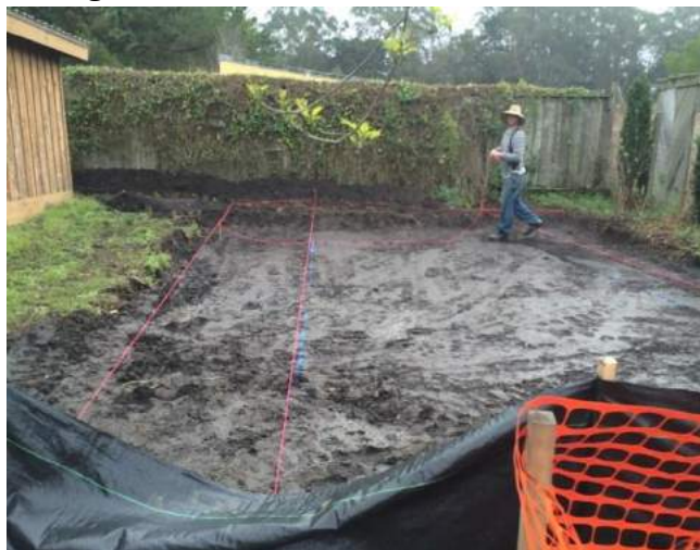
Grading of rain garden and piping installation
