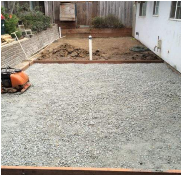
Backyard patio concrete removal and installation of drainage features
