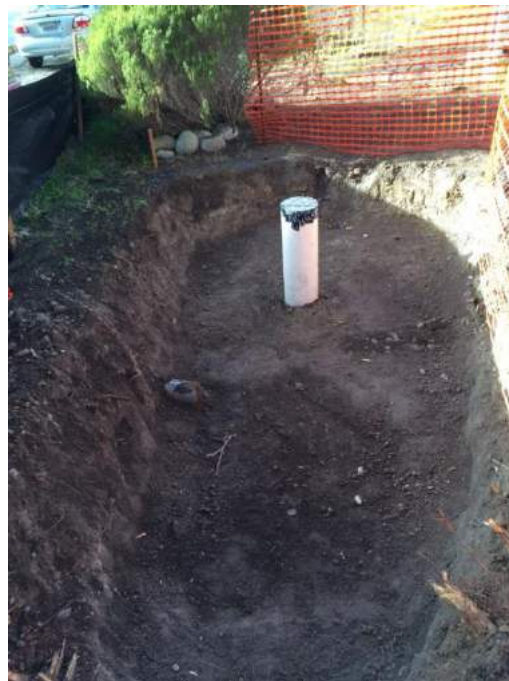
Excavating and laying pipes for western rain garden
