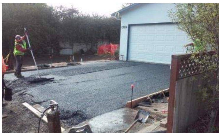
Installation of asphalt driveway with permeable section on top and regular asphalt on bottom
