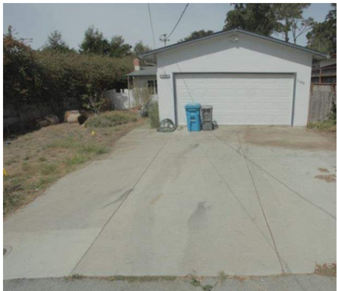
Concrete driveway before permeable asphalt installed Side of driveway to be removed and vegetated
