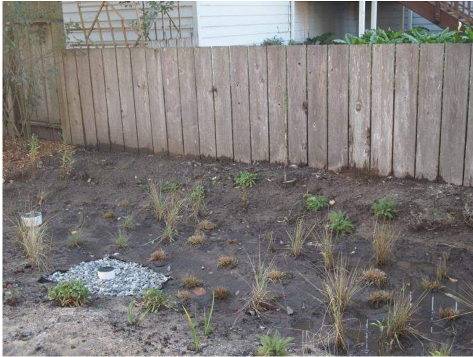
Rain garden with runoff from chicken coop roof and shed
