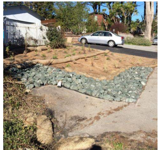
Revegetated side driveway with rain garden drainage outlet and riprap
