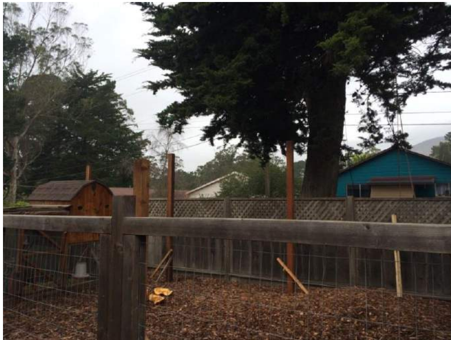
Wooden posts for chicken coop roof structure
