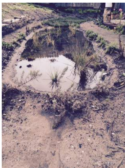
East rain garden after big rain and no-mow sod laid in bioswale which accepts overflow from East Rain Garden
