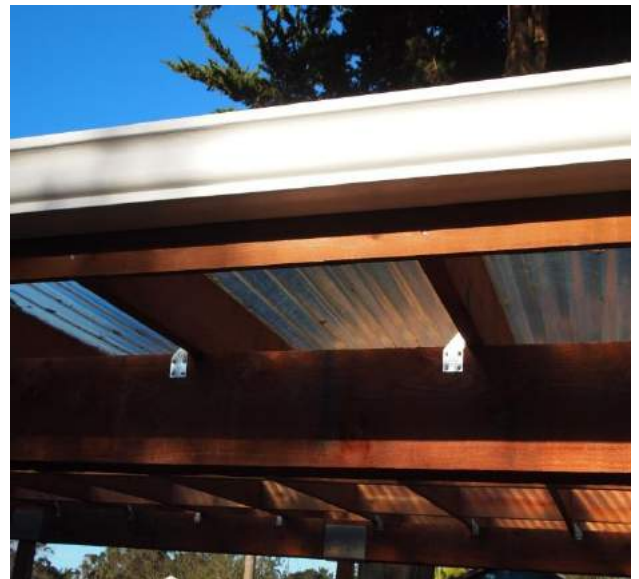
Redwood chicken coop roof with corrugated plastic panels and gutters
