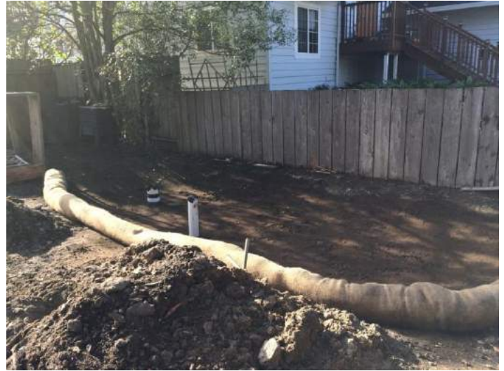
Rain garden installation with piping from shed and around to south side of property
