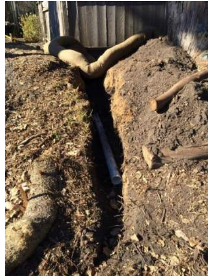
Trench for drain line from rain garden (left) that leads to gravel drainage outlet at road (right)
