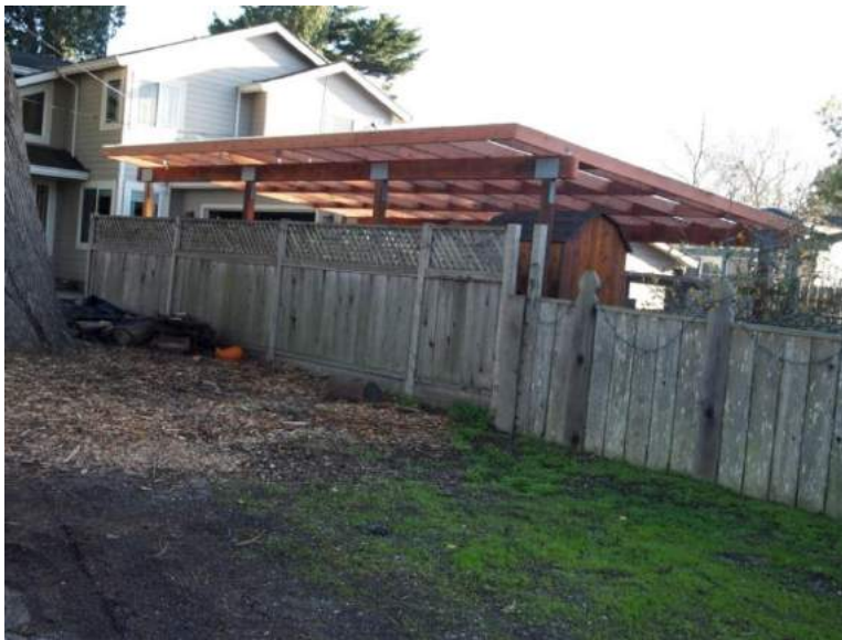
Redwood chicken coop roof with corrugated plastic panels and gutters
