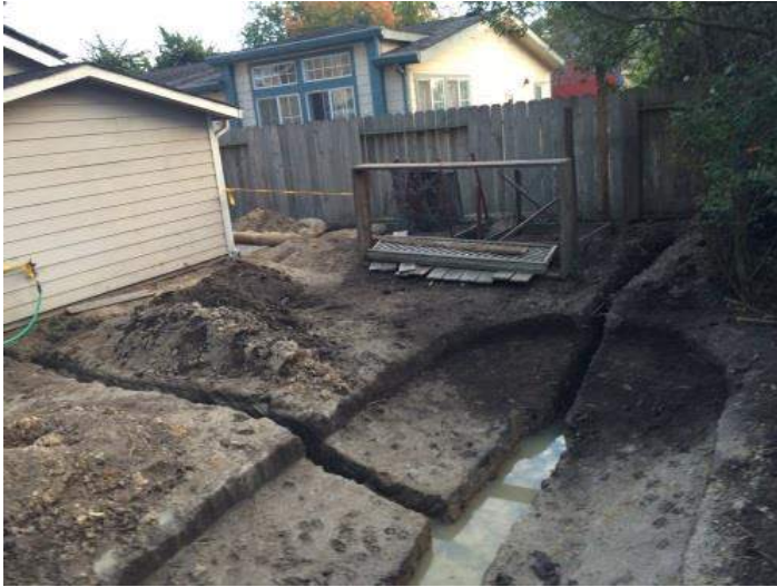
Rain garden installation with piping from shed and around to south side of property
