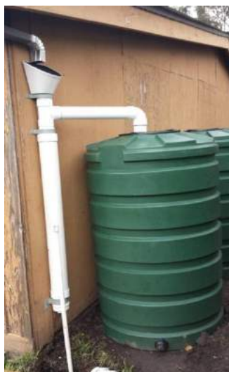
Rain barrels with first flush system
