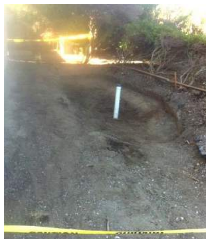
Rain garden area where tree was removed (left), bioswale leading to the rain garden (middle), and bioswale to rain garden connection
