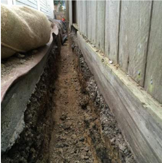
Trench for drain line from rain garden (left) that leads to gravel drainage outlet at road (right)
