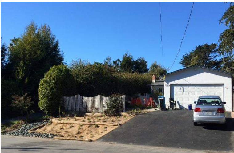
Revegetated side driveway with rain garden drainage outlet and riprap
