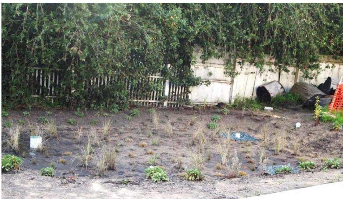
Rain garden with overflow from tanks, and drainage from backyard, north side yard, and driveway
