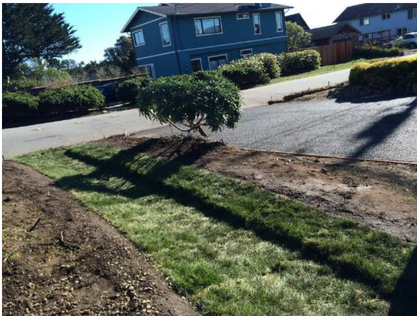
Bioswale with sod (left) and connection of the swale and rain garden (right)
