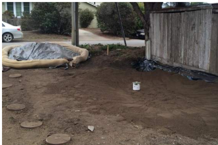
East rain garden installation
