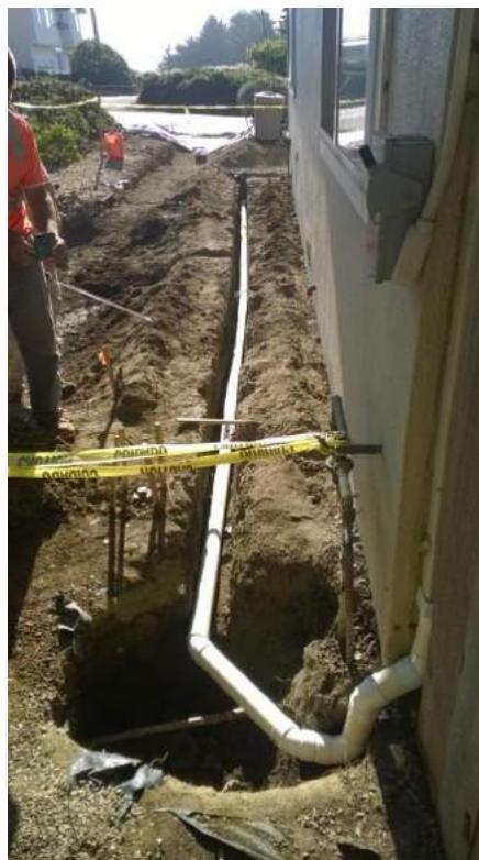
Piping from downspouts to rain garden
