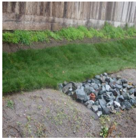
Bioswale leading to three-tiered rain garden system
