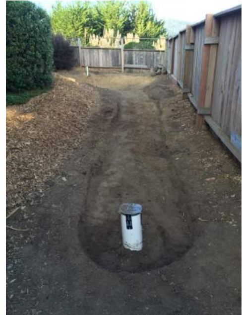
Downstream section of bioswale/rain garden system
