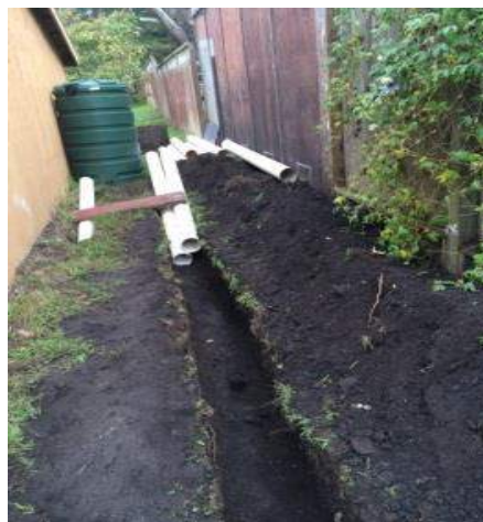
Installations of rain barrels with overflow drain line leading to rain garden
