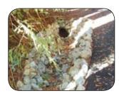
**D** A rocked or vegetated swale lining the edge of a road or driveway reduces erosion potential by SLOWING runoff and then SINKING it back into the soil or directing it to a safer outlet (page 29).
