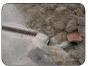
should also be angled at 30-45 degrees. Although slotted channel drains may be installed on any driveway, they are recommended for driveways with slopes greater than five percent.
