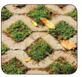
**B** Turf block works well for allowing water to SINK into the soil in medium-traffic areas or driveways with separate parking areas (page 30).
