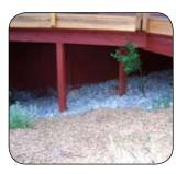
**B** Adding drain rock SLOWS runoff and safeguards the dripline area under elevated surfaces. Mulch around the perimeter adds extra protection to the surrounding bare soil (pages 22-23).
