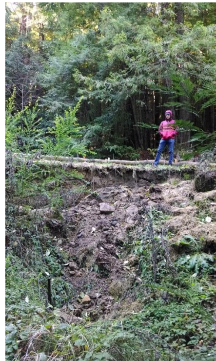
Figure 3. Example of crossing failure: a sinkhole collapsed on the downslope side of Dark Gulch crossing (2015).
