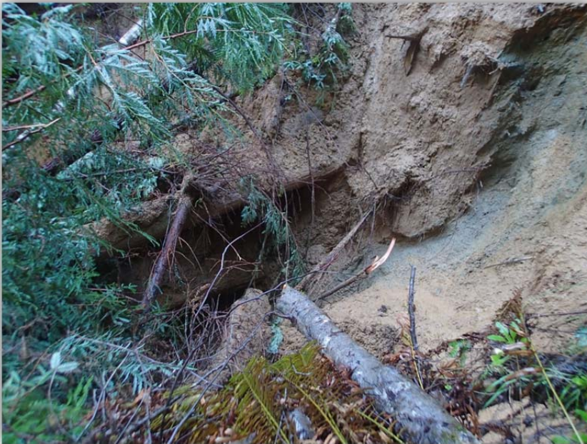
Photo 5 Photo showing lower portion of the 2017 slide scar. The cribwall that had supported the fill embankment is to the left of the photos. The exposed logs are the tie back logs that extended back into the fill prism and proving the structural integrity to the cribwall. With these logs now exposed the structural integrity if the wall has been compromised.
