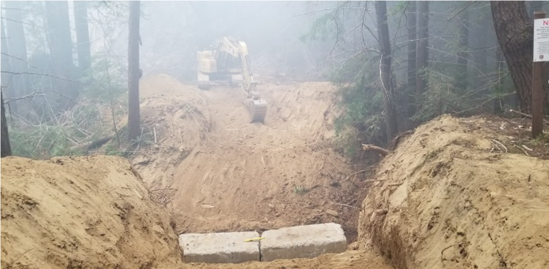
8/25 (Tuesday): Trestle Creek Bridge: Dragging the bridge back into place onto the new abutments.
