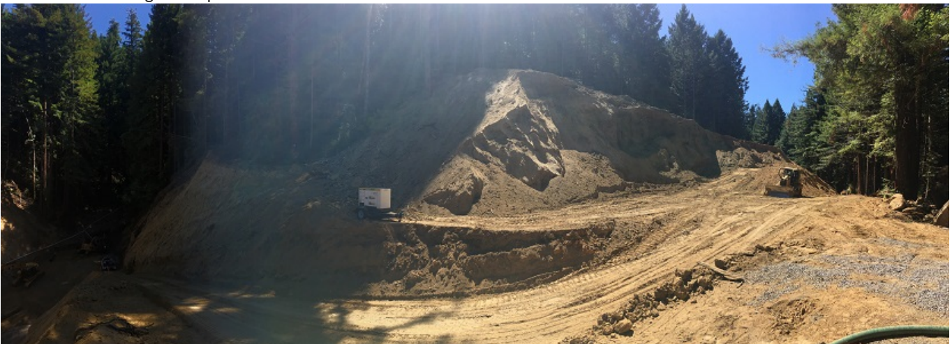
The stockpile of excavated material adjacent to the crossing (on the “bench”) continues to diminish as the crew is using the material to build the crossing back up.
