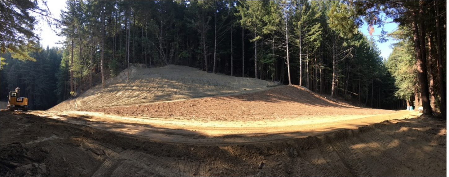
Excavator working on reshaping the road (east of Dark Gulch crossing) for proper drainage of stormwater.
