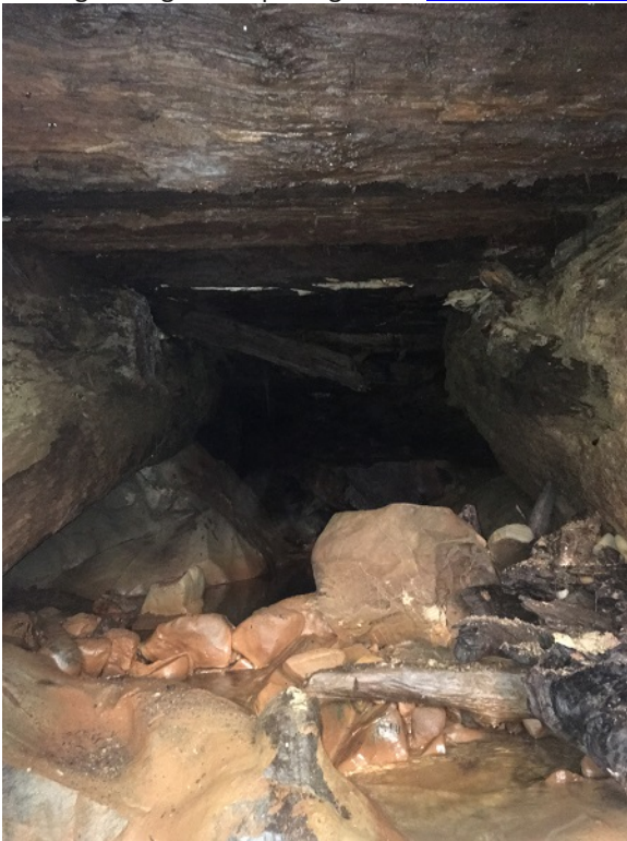
View inside the crib log structure, looking upstream. It looks like a very narrow mine shaft. (Check out the Week 8 video of the water flowing through this opening at the Dark Gulch Construction Gallery .)
