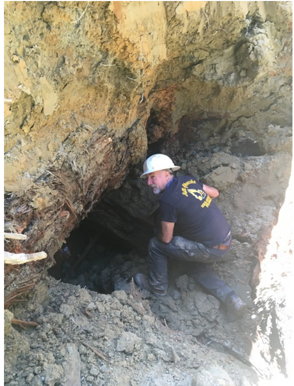
Lester Giacomini (owner, construction company) takes a closer look at the opening to original crib log structure...
