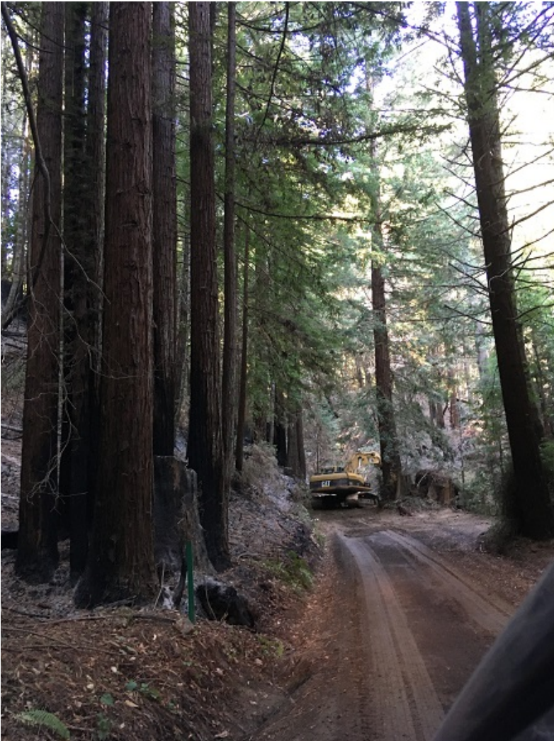
Excavator working on reshaping the road (east of Dark Gulch crossing) for proper drainage of stormwater.
