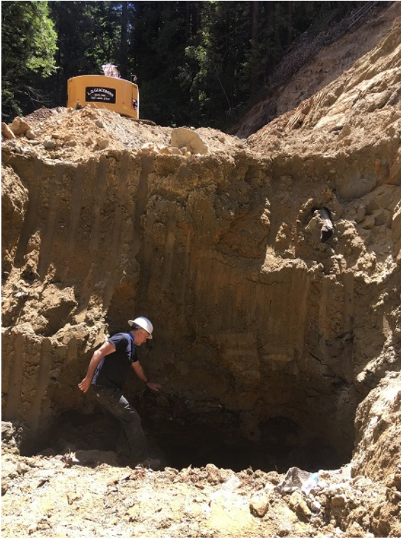
Opening to original crib log structure...
