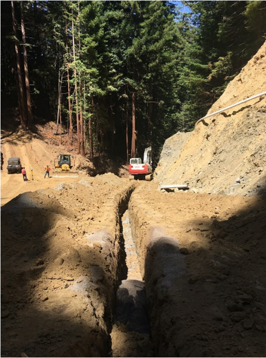
Looking downstream at the trench for one of the subdrains.
