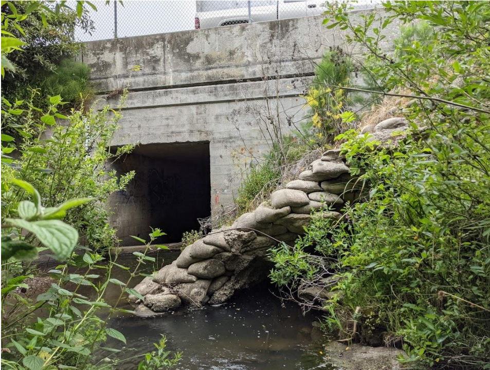
Photo 1: Adobe Bridge culvert inlet and failing sac-crete revetment (May 2021).
