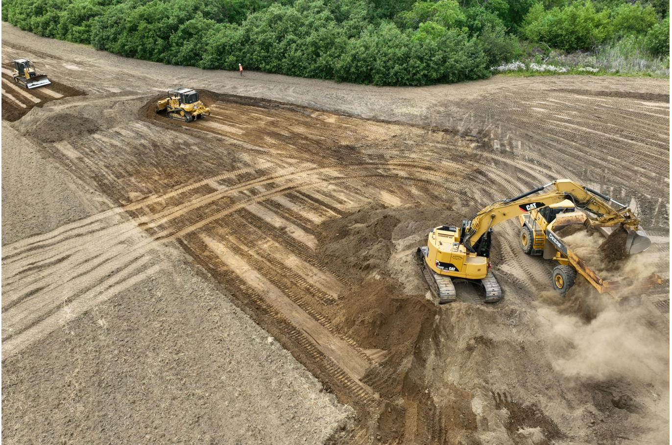
Excavators creating floodplains at the Butano Creek project site (Photo: San Mateo RCD)
