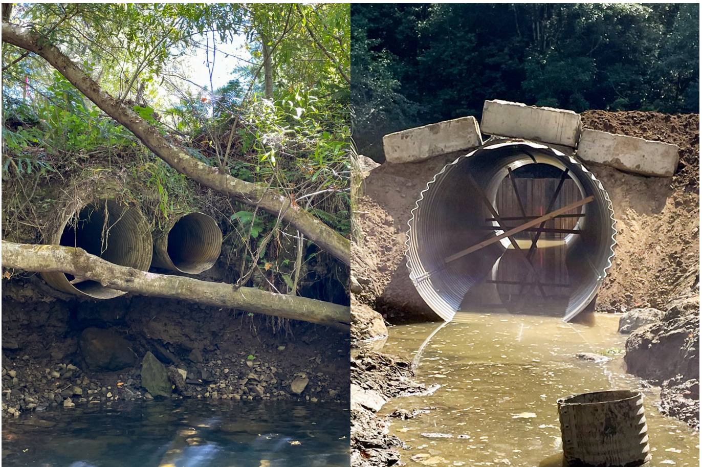
Original culverts at the Dry Dock Gulch site (left) versus the new culvert (right). (Photo: Trout Unlimited)
