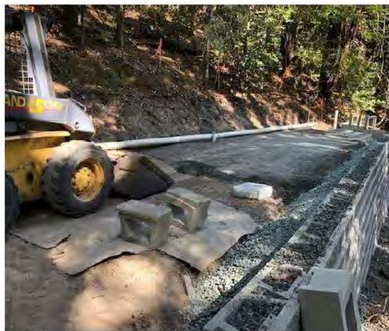
Construction of retention wall & tank pad
