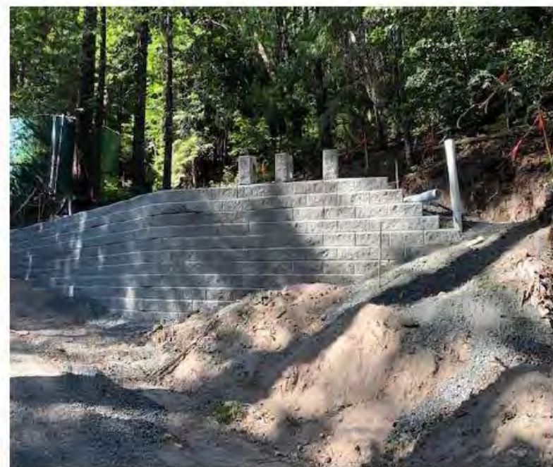
Construction of retention wall & tank pad
