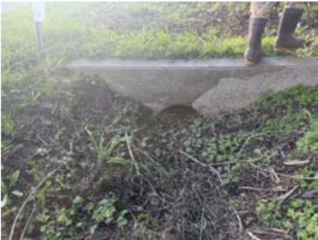
Photo 9: Stormwater conveyance towards Butano Creek on southern border of the Subject Property
